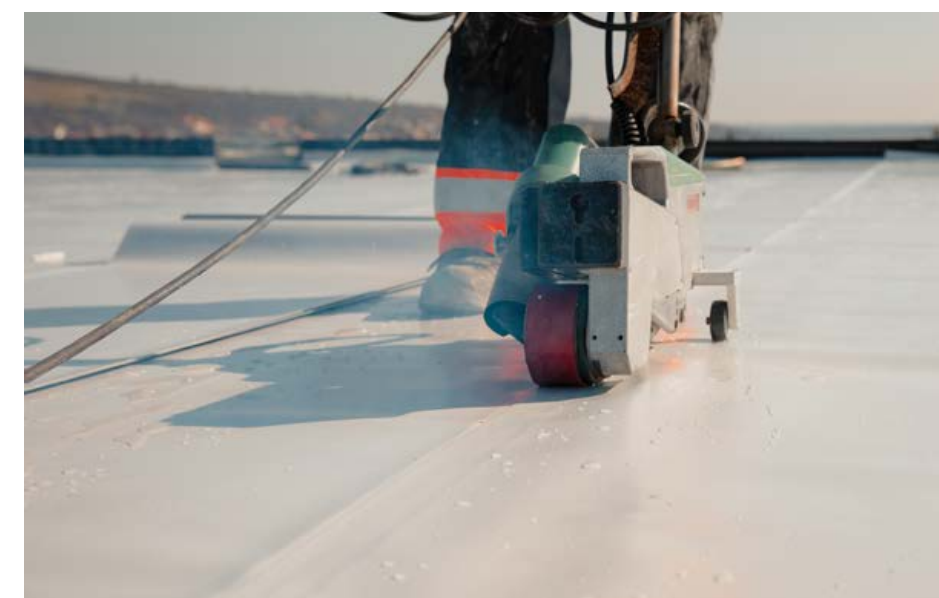
Thermoplastic polyolefin roof
